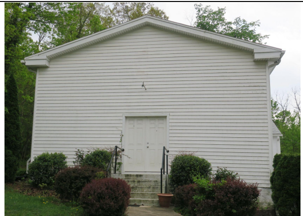
d) Town Hall (formerly St. Mark's Methodist)
